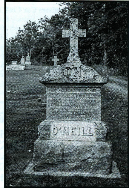
A few years ago, Campbell Monument of Belleville offered to repair old/damaged gravestones at several cemeteries in the Central Hastings area at a greatly reduced cost. This is one of the excellent repairs, to the monument of Captain John O'Neill in Sacred Heart Cemetery. Photo by Emily Winowich
